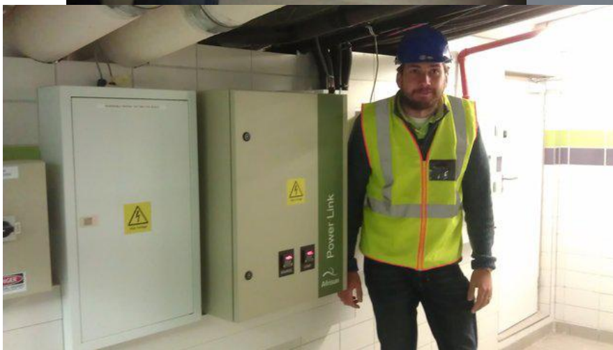
Pictures 7a/7b/7c: Hotel Verde, Cape Town, 70kW Grid-tie solar inverter
