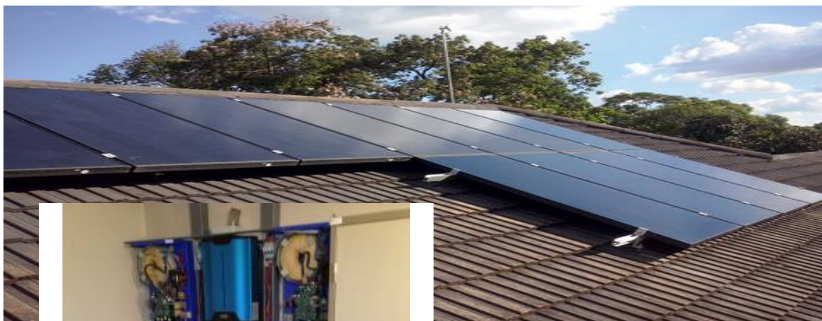
Picture 1: Roof mounted solar panels. Note the proprietary aluminium mounting system. This keeps the panels raised from the roof allowing cooling from behind and also allows leaves and debris to wash through.
