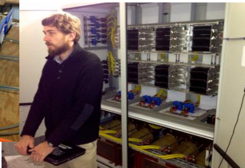
Pictures 6: Neil working on 500kW grid-tie solar inverter
