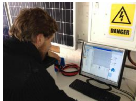
Picture 4: Neil working on solar system SCADA software
