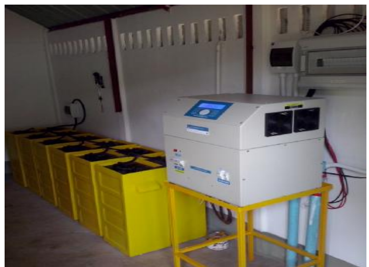
Picture :12 Inverter room after construction during electrical installation
